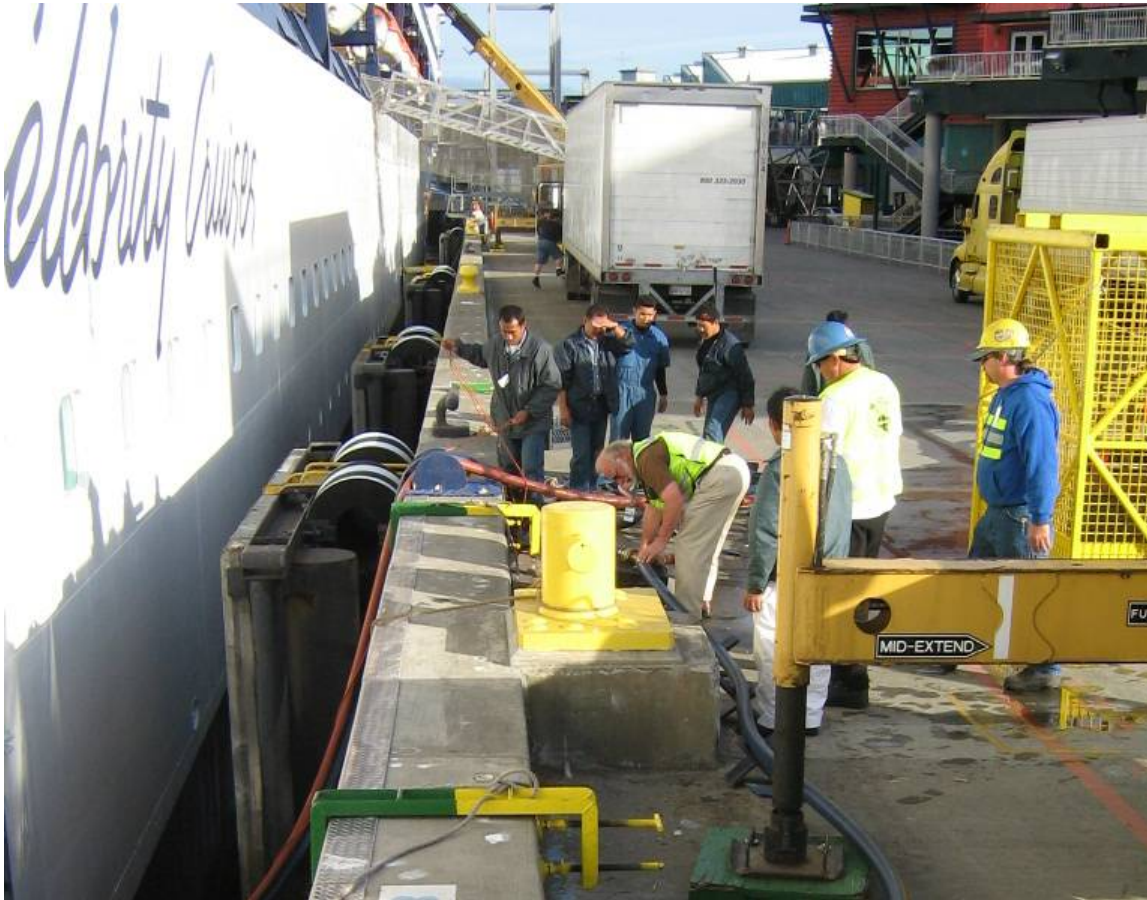
Figure 19. Pier Access (Pier 66)
