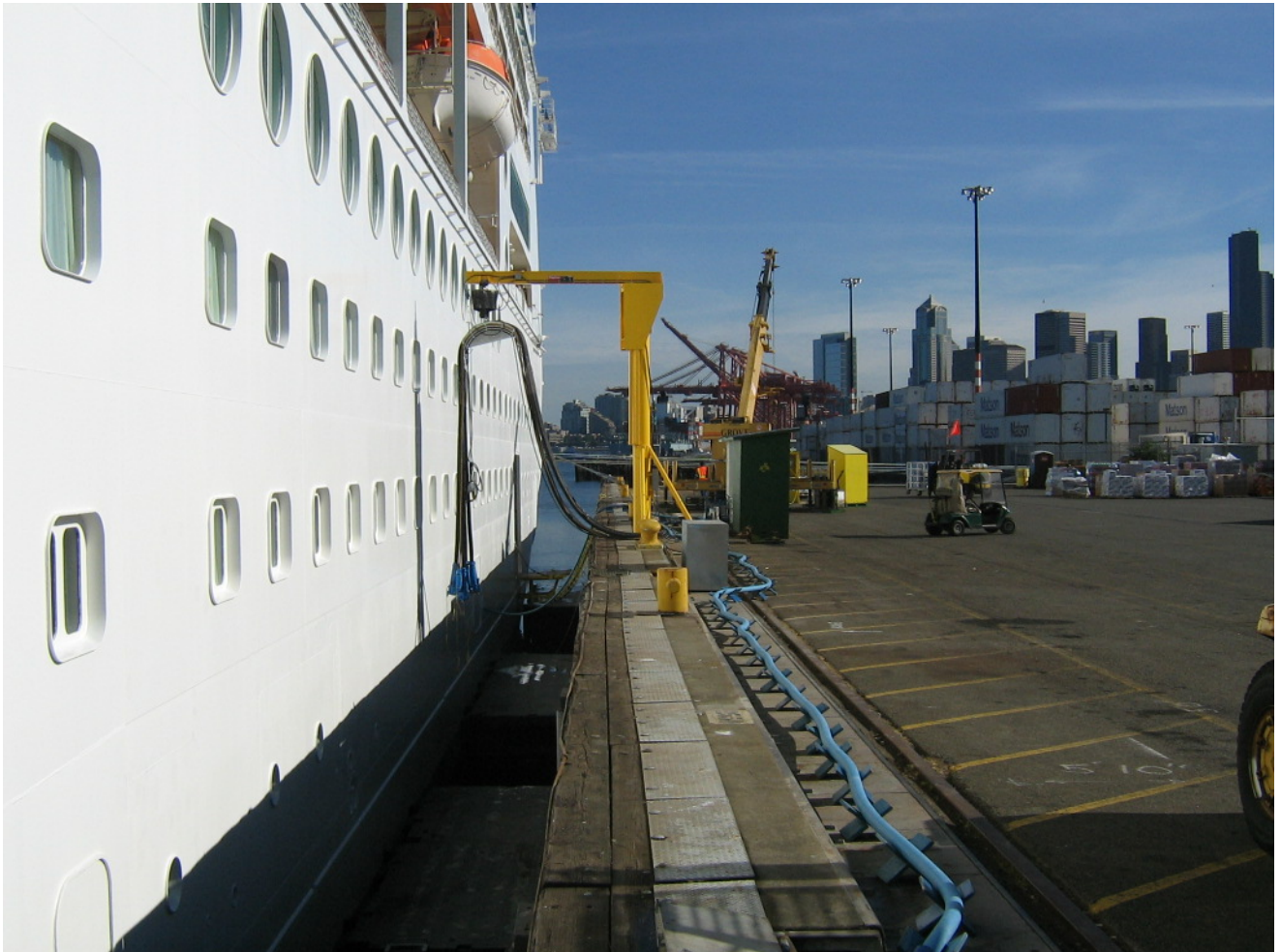
Figure 17. Vessel Shore Power Connection (Terminal 30)
