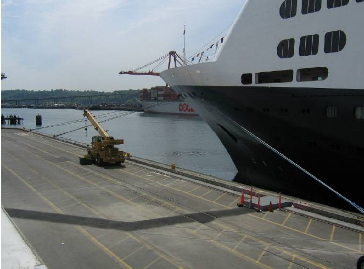
Figure 10. Vessel Mooring Lines (Terminal 30)
