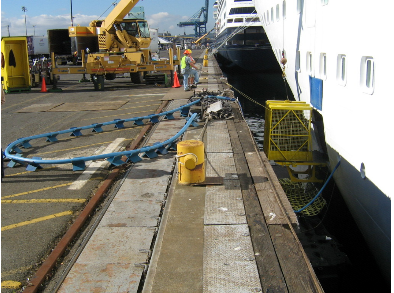
Figure 16. Utility Connection (Terminal 30)
